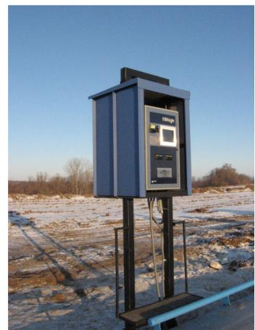
A thermostatically controlled heater unit assures the internal temperature of the enclosure remains warm even though the Iowa wind chill often reaches -20 degrees below zero.
